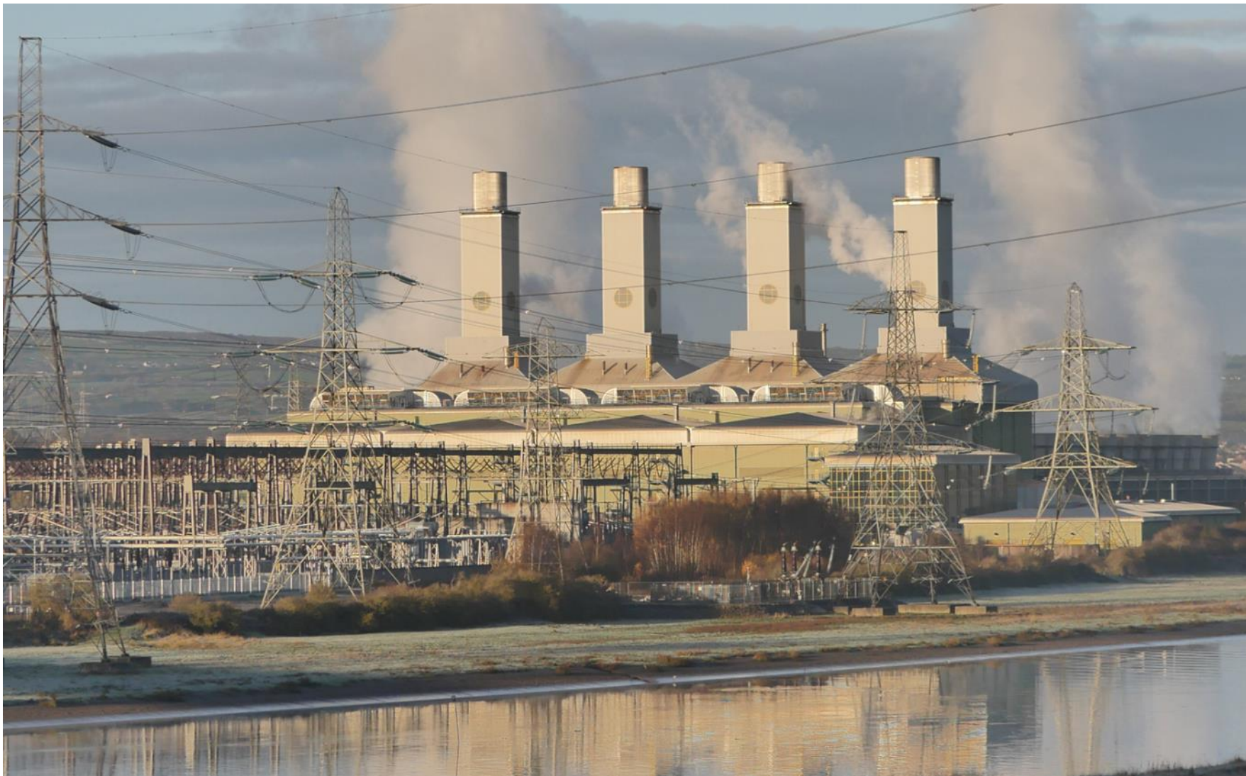
Plate NTS 10: Existing Connah's Quay Power Station (view from Dee Estuary)
